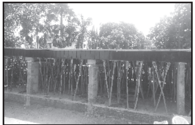
On going project of Prathna hall & Guest House construc- tion at Gandhinagar Temple
